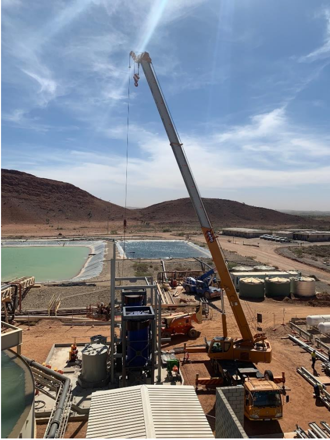
Figure 8: Regrind mills installation
