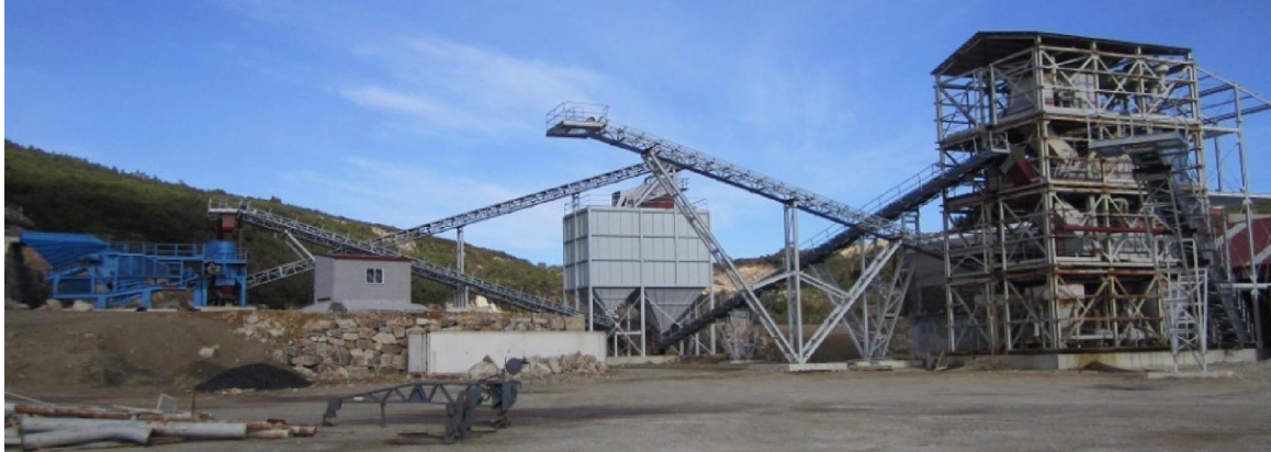
Figure 5. Primary crushing, screening and dense media separation plant constructed in 2012.
