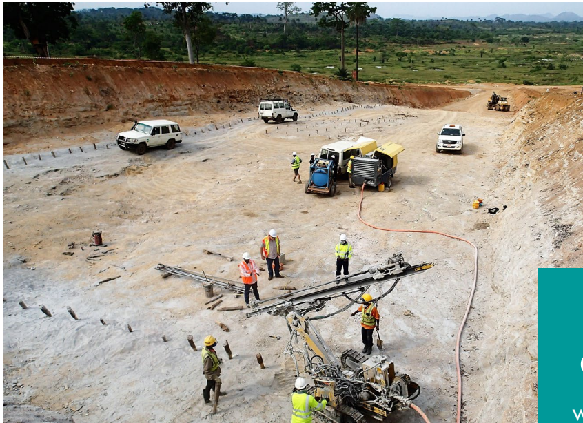
Box cut pre-blast drilling
