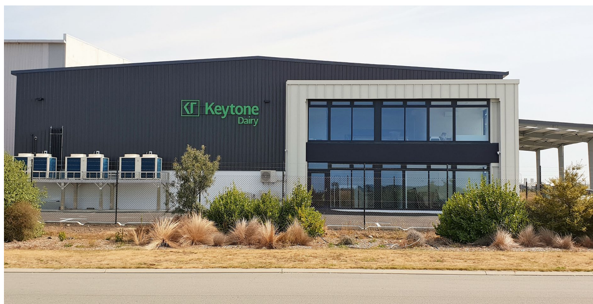
Keytone Dairy's second purpose-built manufacturing facility under construction through FY19
