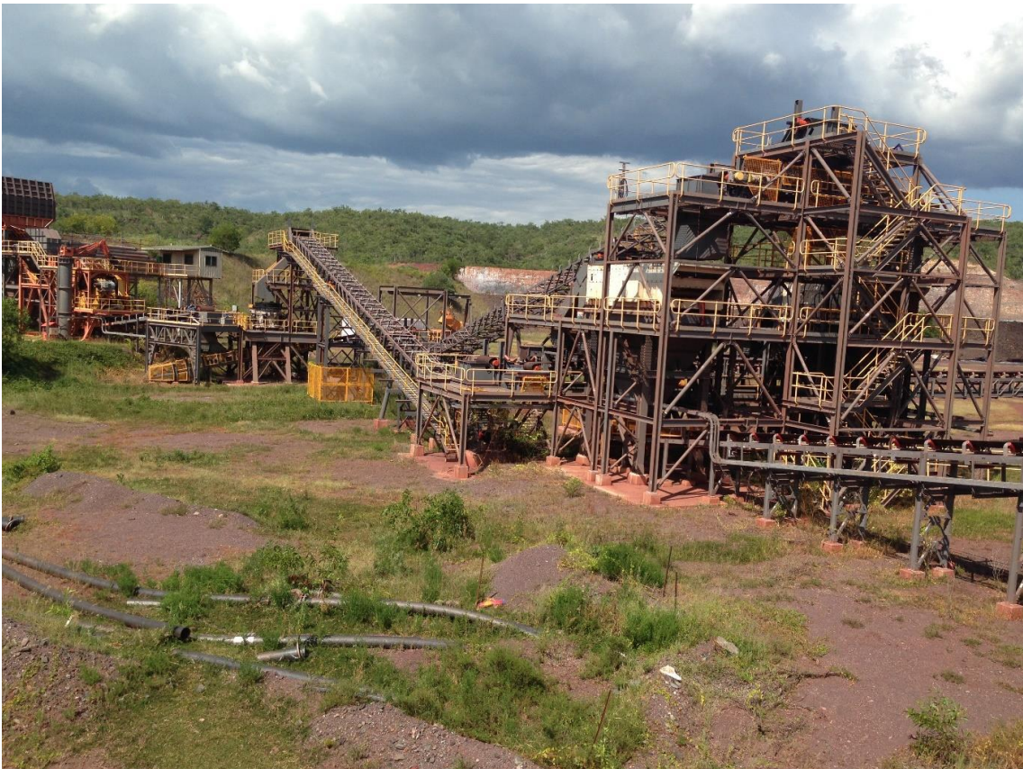
Frances Creek Crushing and Screening Plant
