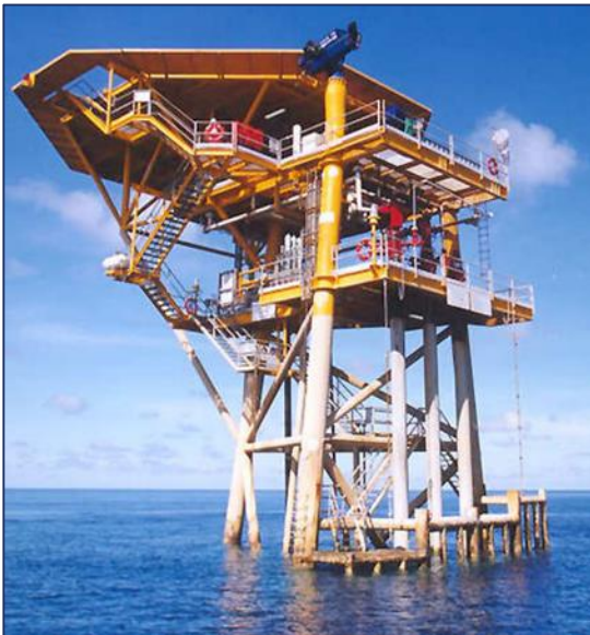
WELL HEAD PLATFORM
