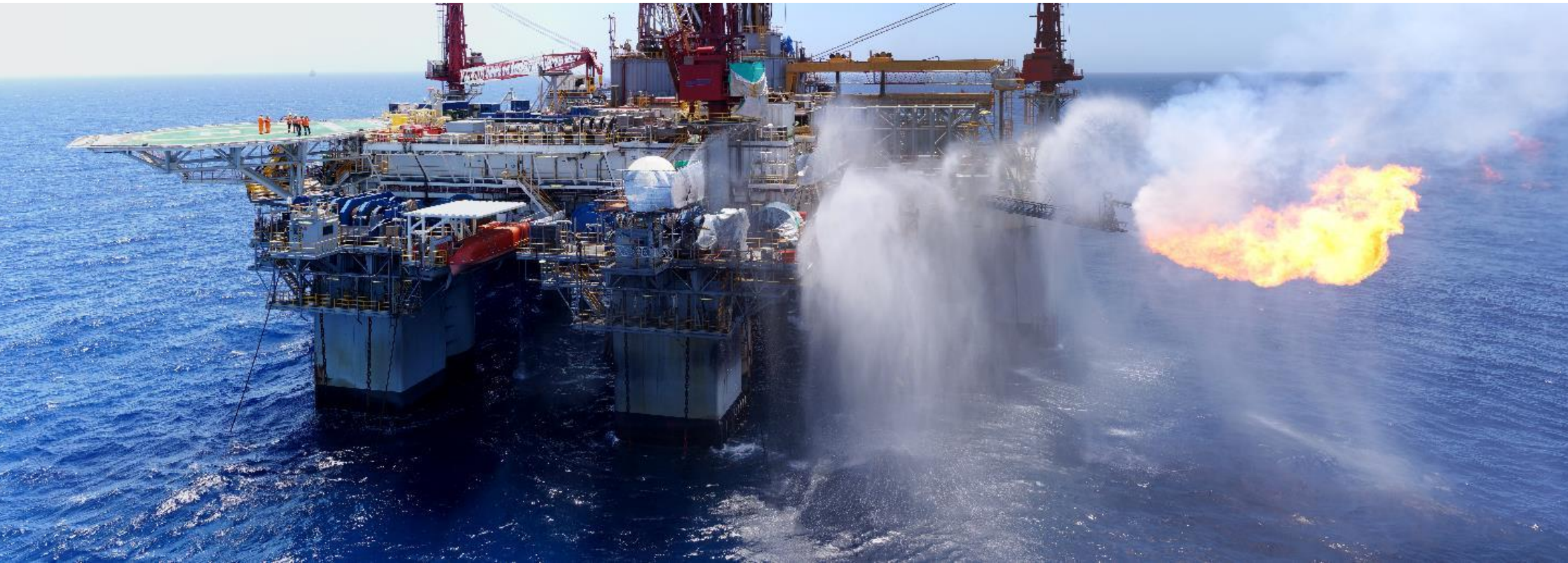
Photo of the Roc-2 well flowing at commercial rates on test in late 2016 Flow rates of 53 mmscf/d and 3,000 barrels of condensate per day were at maximum test equipment capacity The Roc-2 well bore is approximately 20 kilometres from the Dorado-1 well bore (within tie back distance).
