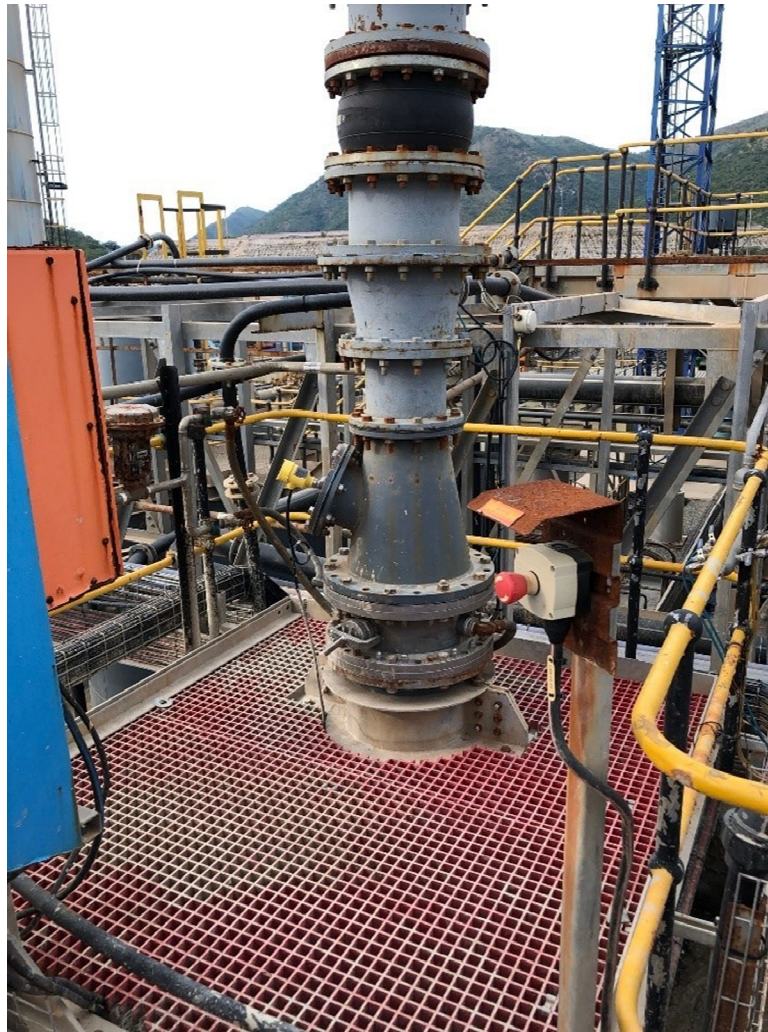
Figure 5: Aachen™ Installation – Gold Mine Example 3
