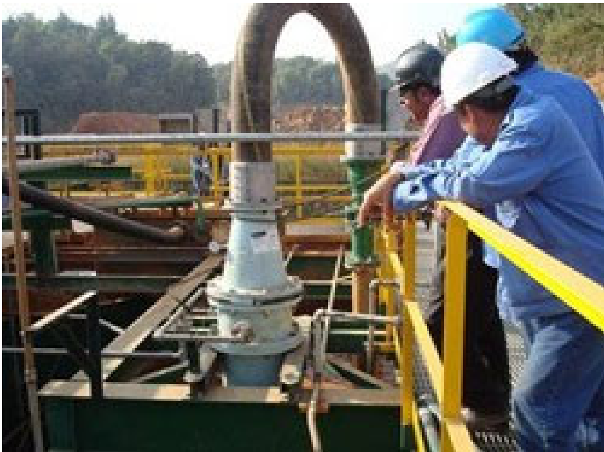
Figure 3: Aachen™ Installation - Gold Mine Example 1
