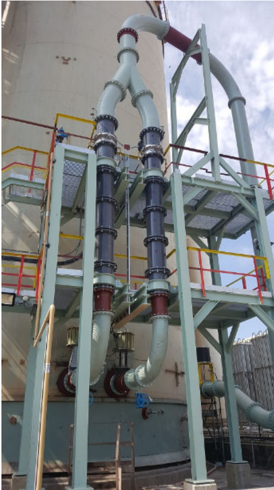
Figure 4: Aachen™ Installation – Gold Mine Example 2
