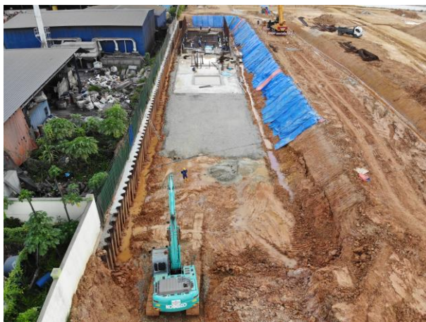
OSD Tank Excavation and Construction Preparation
