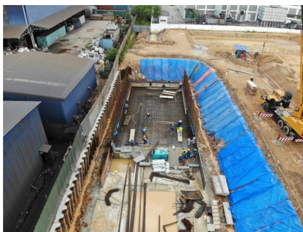
OSD Tank Excavation and Construction Preparation
