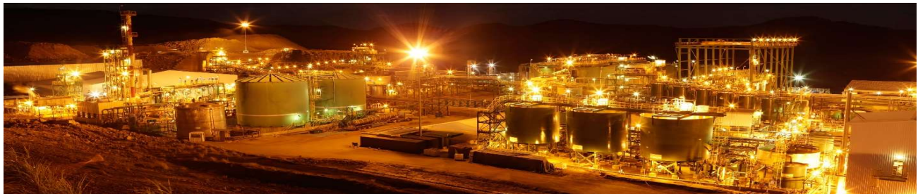
Figure 1: Kayelekera Process Plant
