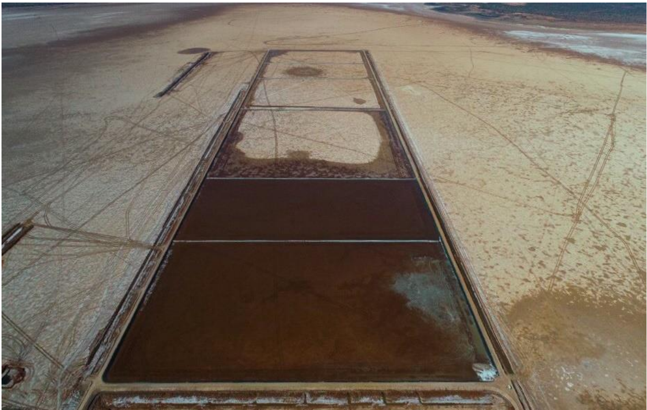
FIGURE 1 BRINE PUMPING INTO EVAPORATION POND
