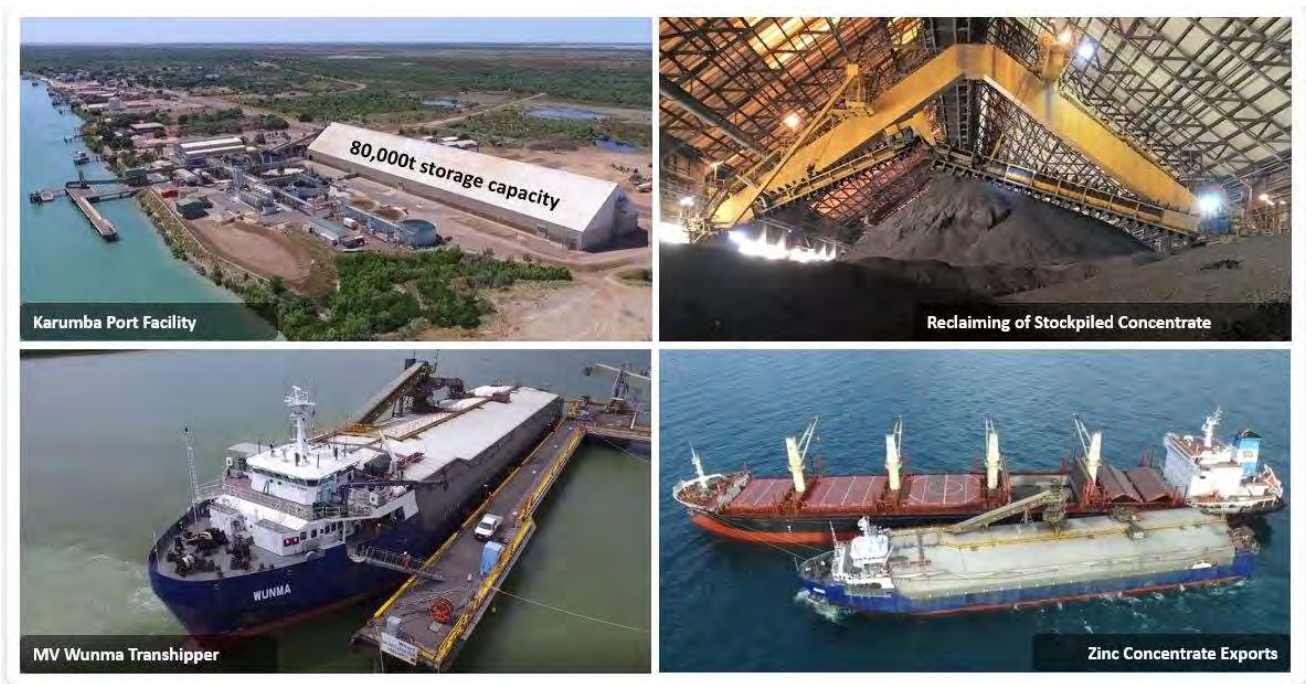
Figure 9: Product logistics infrastructure at Karumba Port Facility
