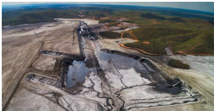
Figure 3: Current progress of hydraulic mining at Lawn Hill
