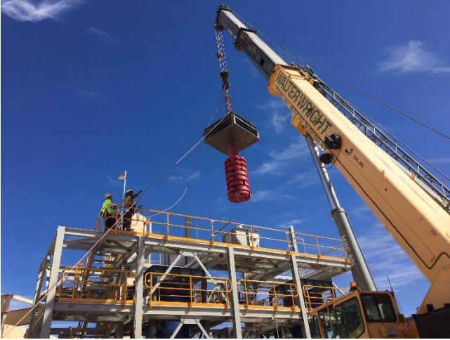
Figure 2: Mill agitator assembly being loaded into the mill shell
