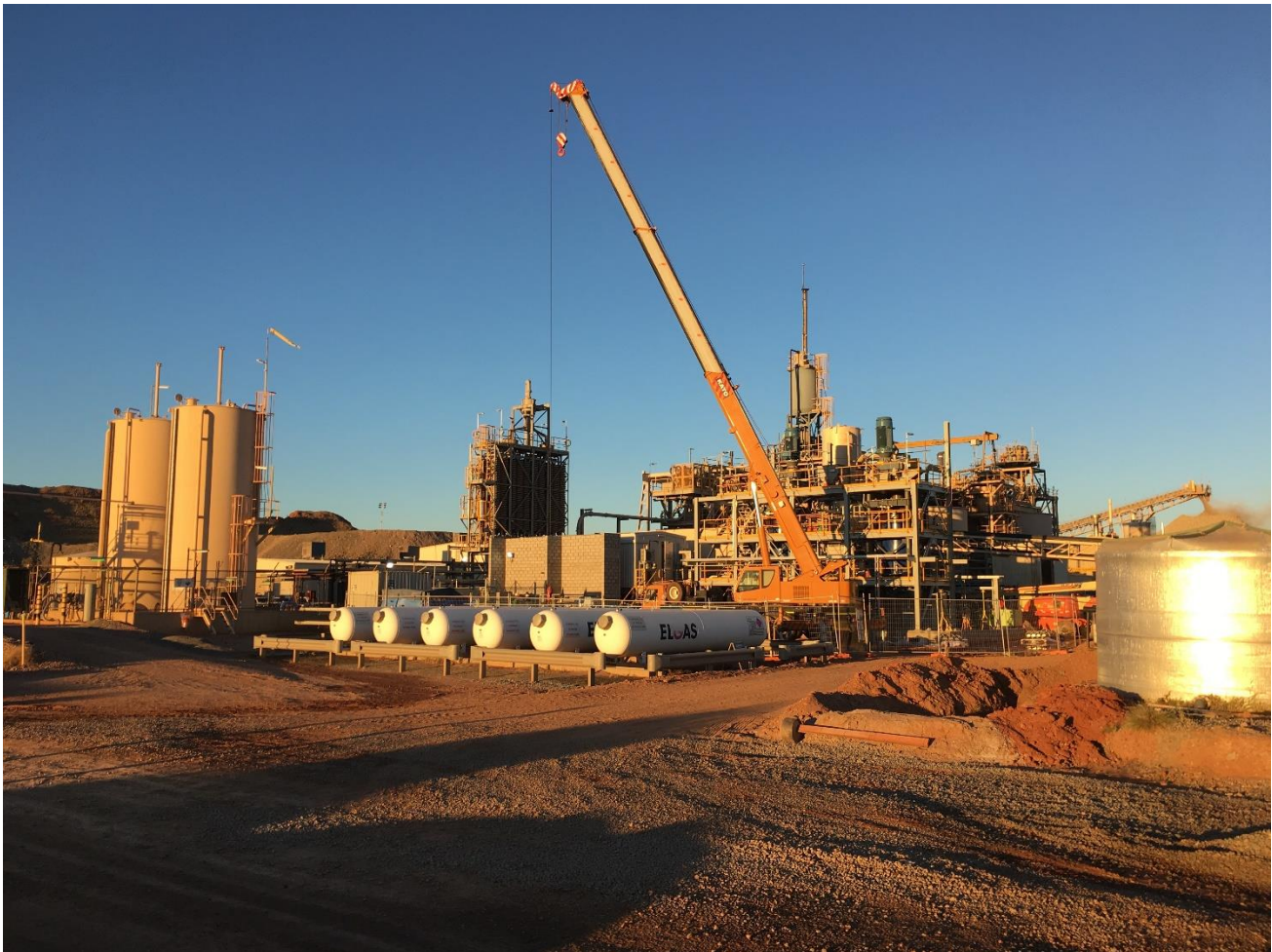
Figure 1: Concentrator and mill area during final stages of construction
