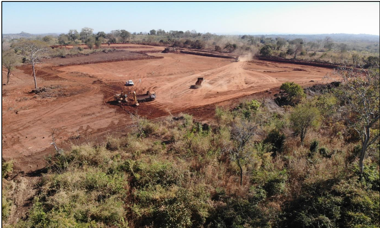
Figure 2: Terracing and Levelling at the Processing Plant Area.
