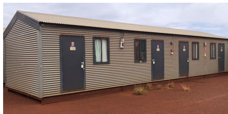
Accommodation Rooms Installation Commenced
