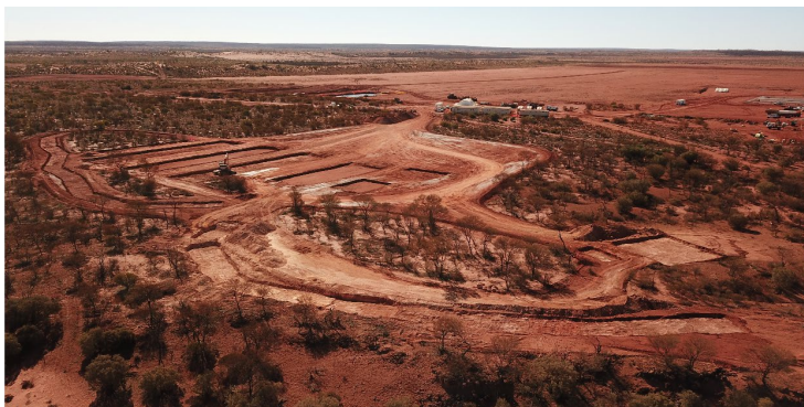
Village Earthworks Complete
