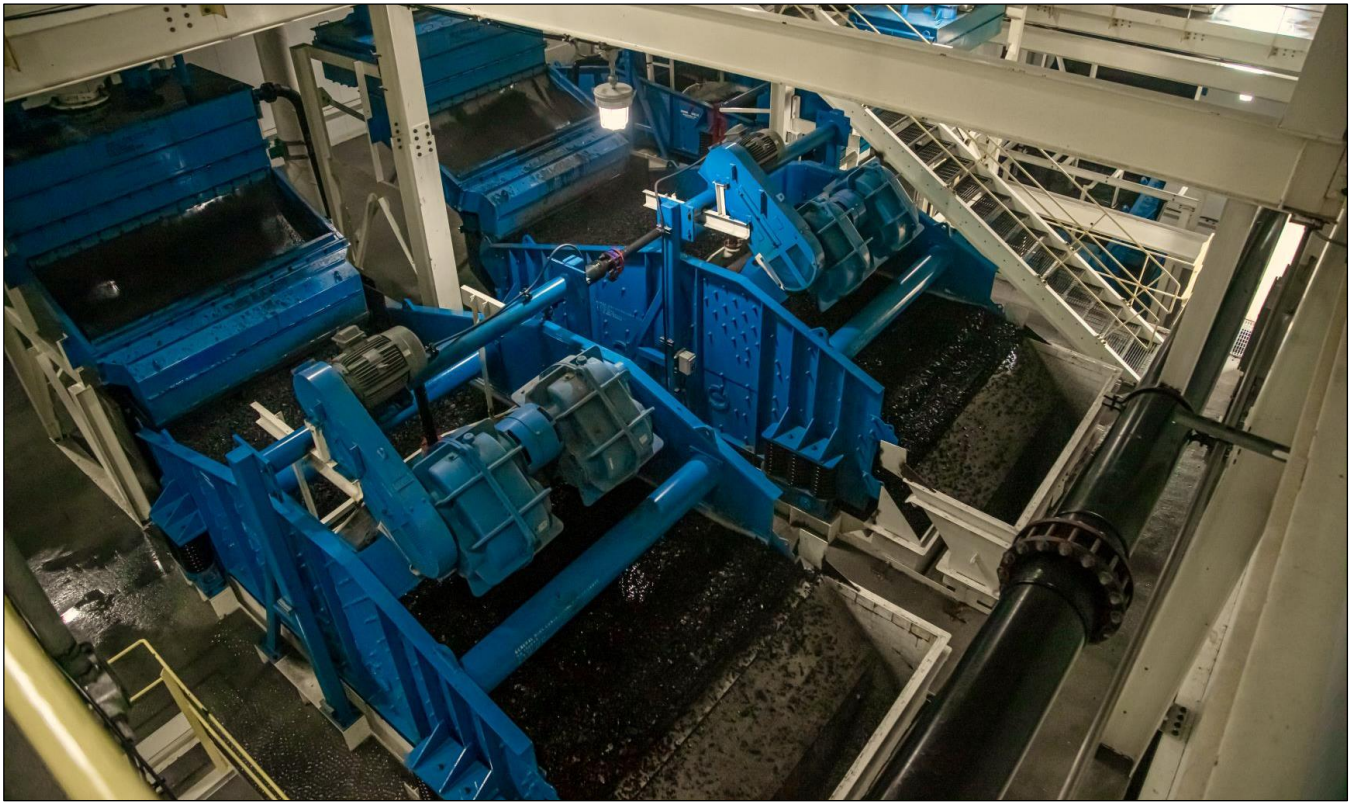
Figure 5: Product screens at the Poplar Grove CHPP
