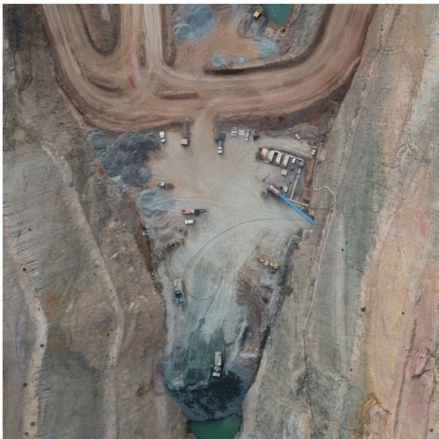
Figure 1: Rosemont UG portal area (South end of Rosemont Main Pit).
