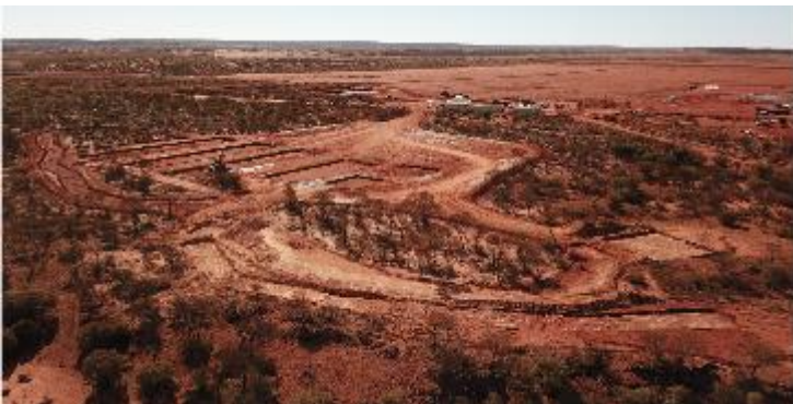
Village Earthworks Complete
