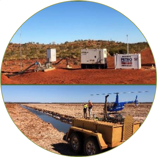
Brine Pumping from Bores and Trenches >260 Million litres successfully pumped to date
