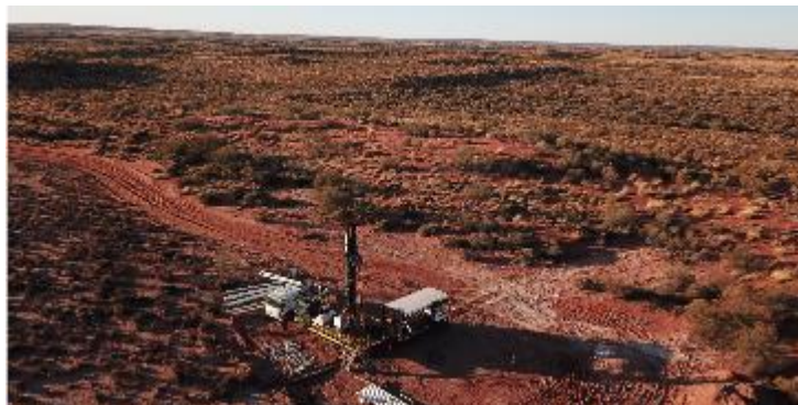
Fresh Water & Brine Production Bore Drilling
