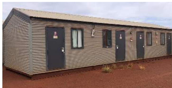
Accommodation Rooms Installation Commenced
