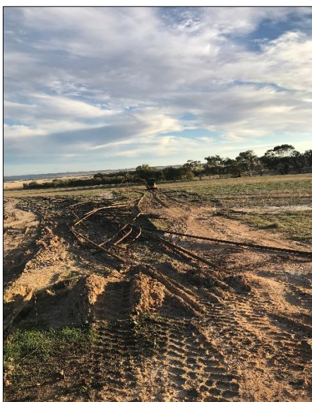
Decommissioned flowline (left) around Mh-7 and Mh-13 with rehabilitation (middle and right)
