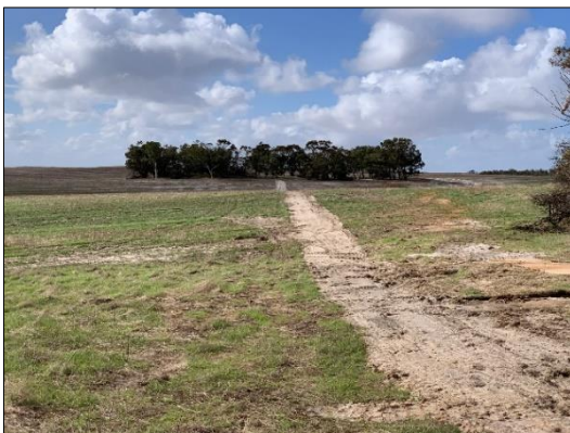
Fully rehabilitated Mh-7 flowline (left) and partly removed and decommissioned Mh-3 flowline (right)
