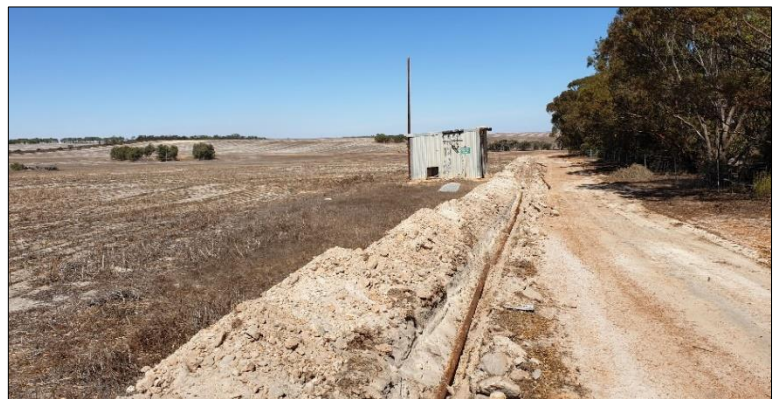
Fully rehabilitated Mh-7 flowline (left) and partly removed and decommissioned Mh-3 flowline (right)
