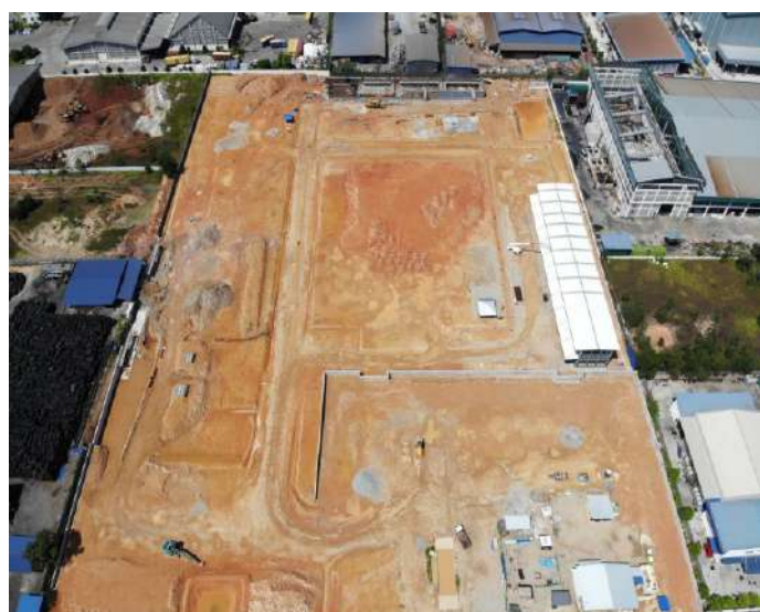
HPA Plant Construction
