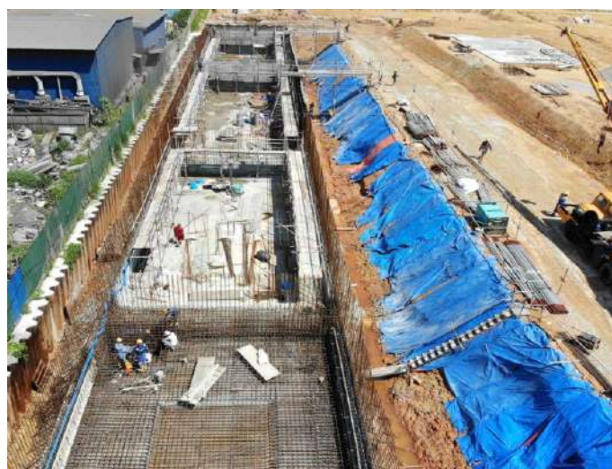
HPA Plant Construction
