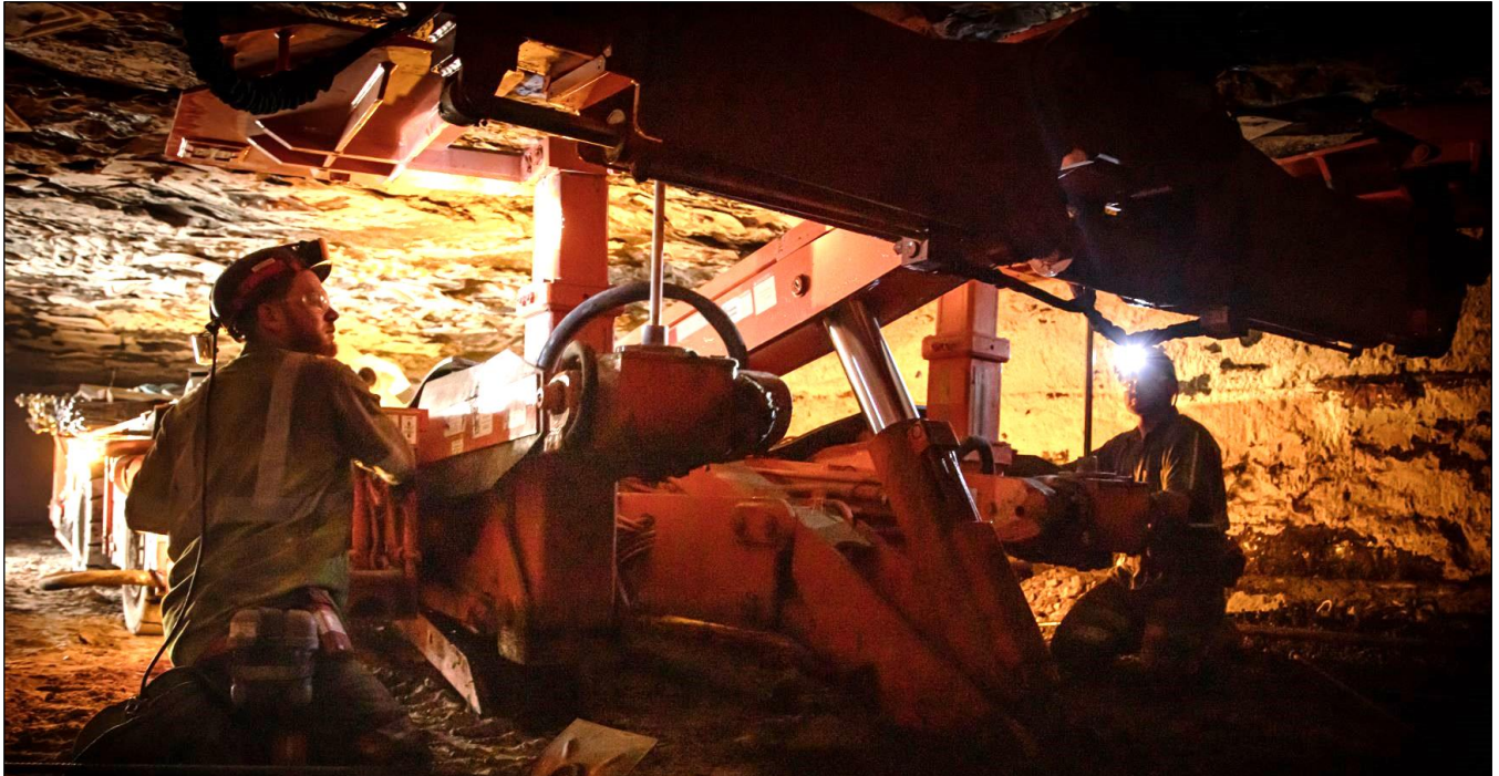
Figure 7: Roof bolting activities at Poplar Grove
