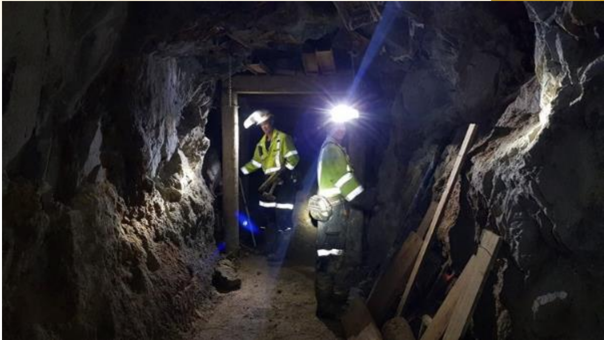
Figure 3 - Timber sets being constructed to reinforce the brow at the entrance to the Dubbo Rise
