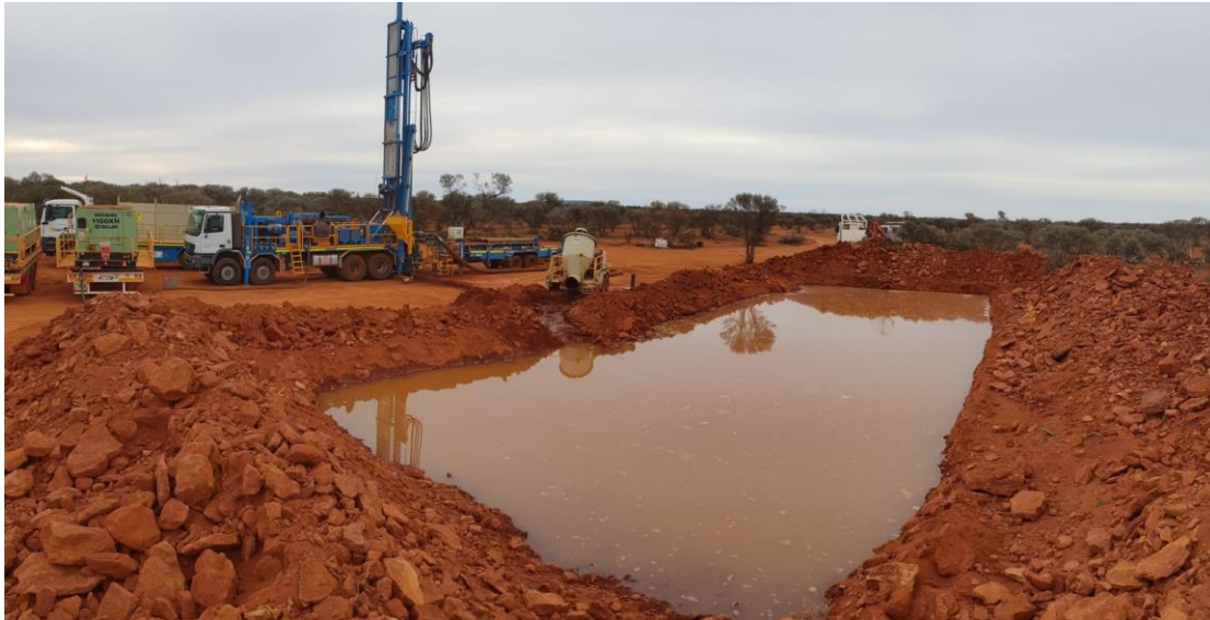
Figure 5 Water resource drilling underway at The Australian Vanadium Project
