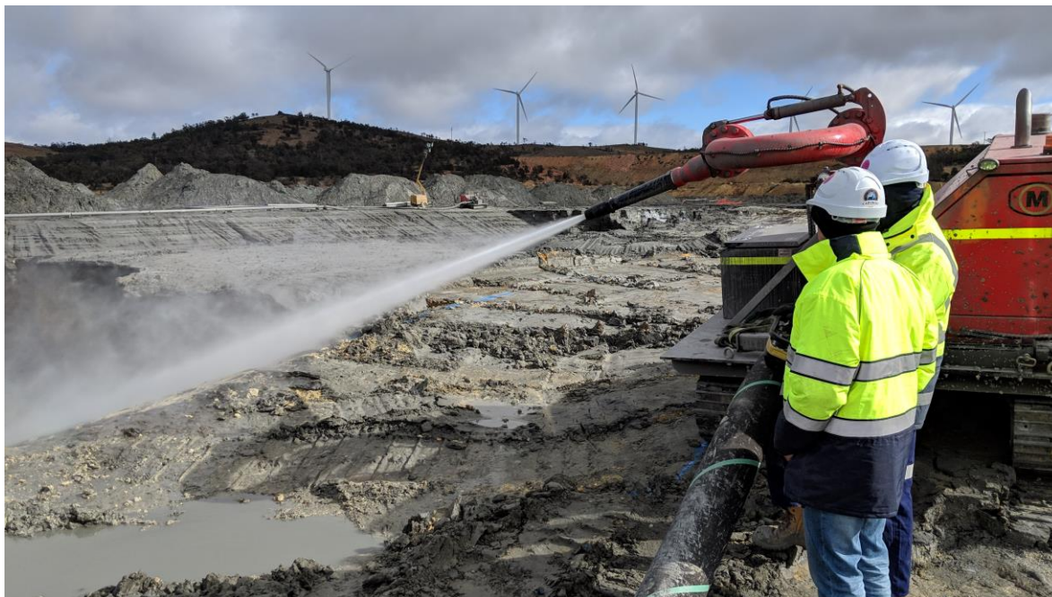
Figure 6 Hydraulic mining progressed through the quarter with completion of the main delivery trench in Tailings Dam South.
