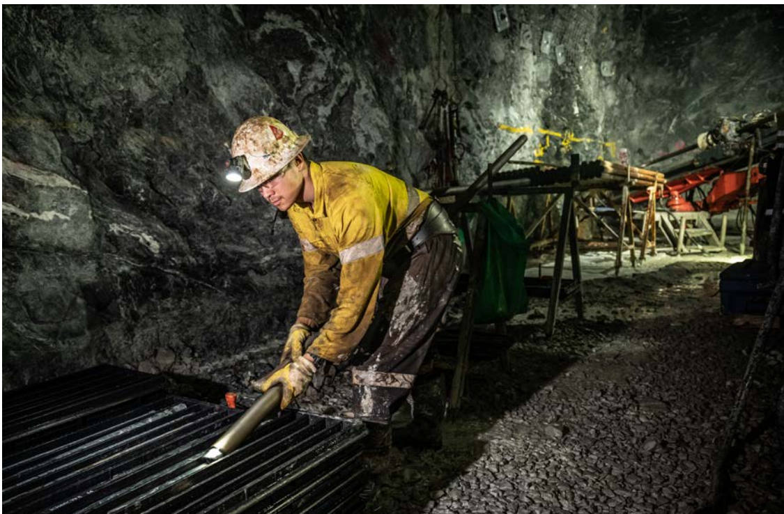
Plate 1: Underground Diamond Drilling operations.
