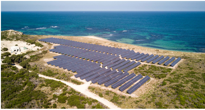
Figure 2 - Garden Island Microgrid Project - A 2MW solar PV installation and 2MW/0.5MWh battery energy storage system.
