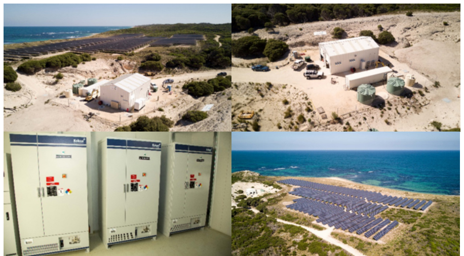
Figure 6 - clockwise from top left: array looking north with battery building in foreground; desalination container and tanks in foreground; array looking west out to offshore wave energy area; battery banks in climate controlled room.
