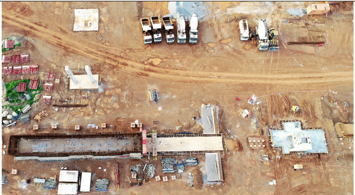
Photo 5: Reclaim tunnel and pebble crusher pad.
