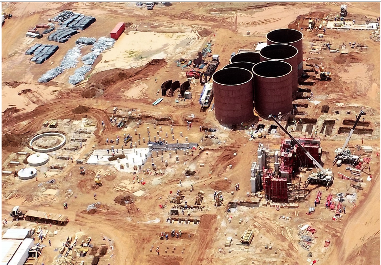
Photo 2: Process plant area. CIL tanks, milling and thickener areas.
