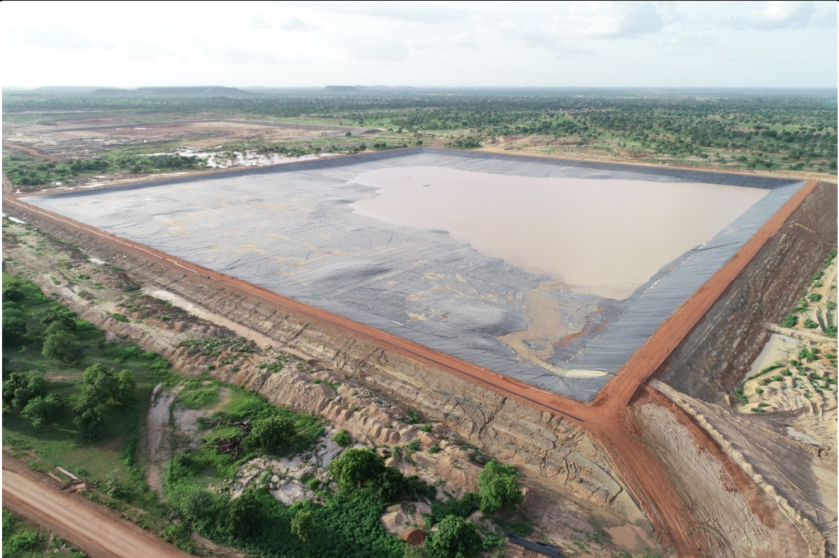
Photo 3: 500m x 500m lined 1.5M m 3 WSF. Pumping in progress see bottom right corner.
