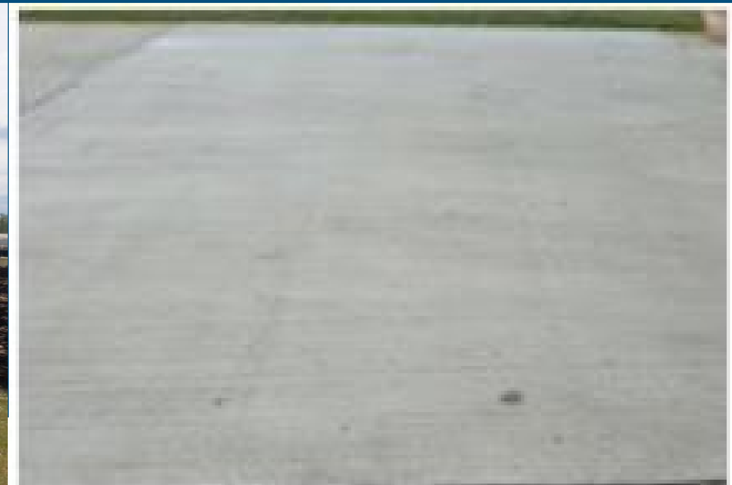
EdenCrete® TRIAL SLAB
