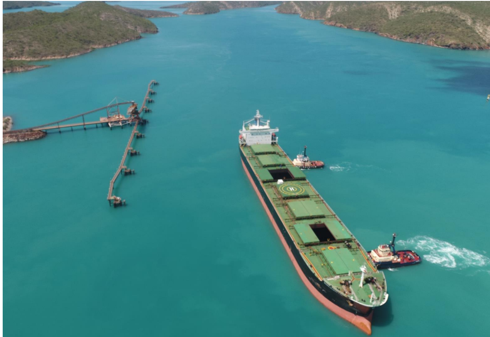
Bulk carrier berthing at Koolan wharf, April 2019
