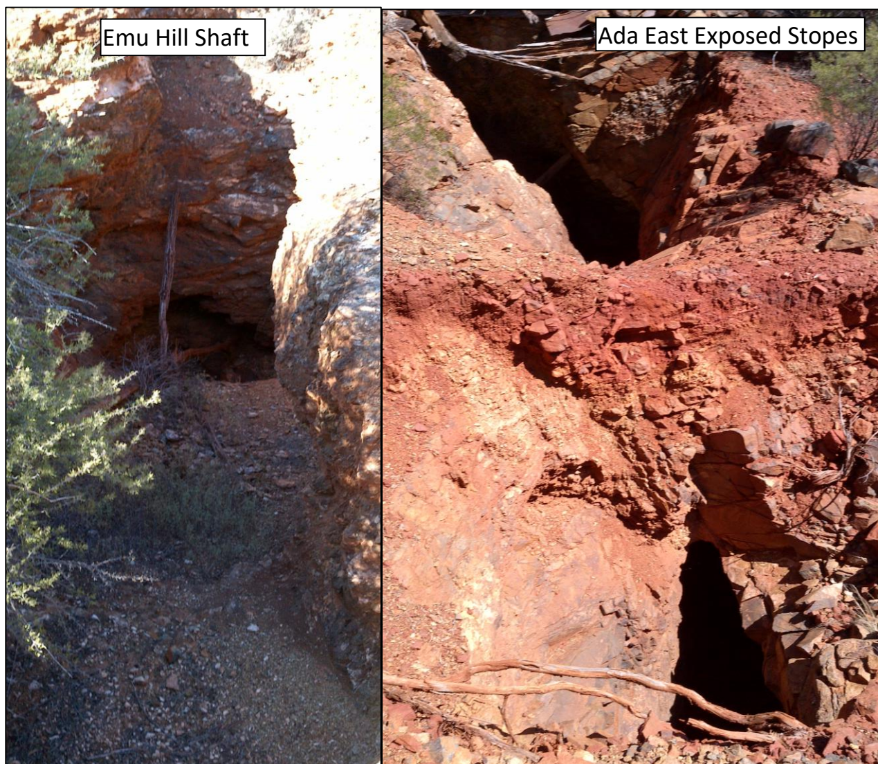
Figure 3: View south of shaft at Emu Hill and view of NW open stopes at Ada East
