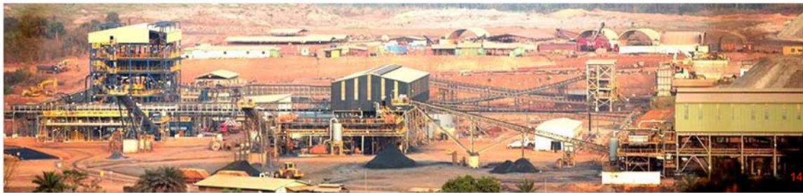
Figure 5: An Overview of the Marampa Mine Processing Plant
