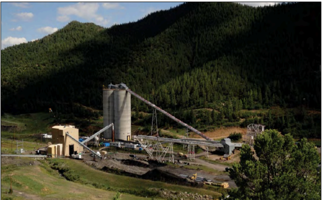
Image: Aerial view of the New Elk Coal Mine today: ROM and Product pads; CHPP; and twin storage silos.
