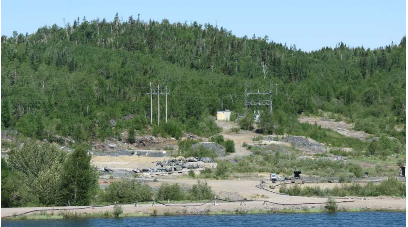
Image 11: Plant Site and Power Infrastructure
