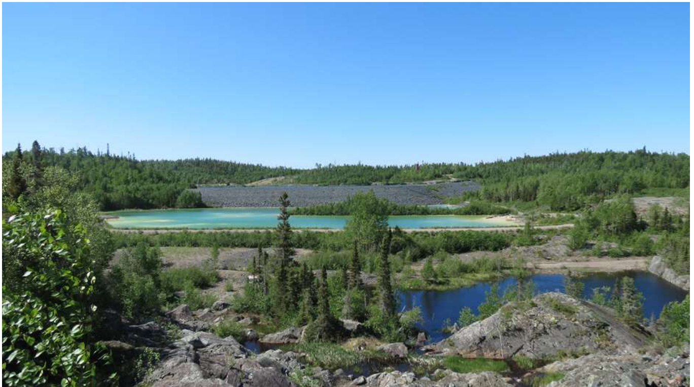
Image 10: Tailings Storage Facility from Plant Site
