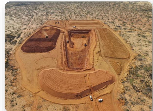
Test Pit Free Dig Mining
