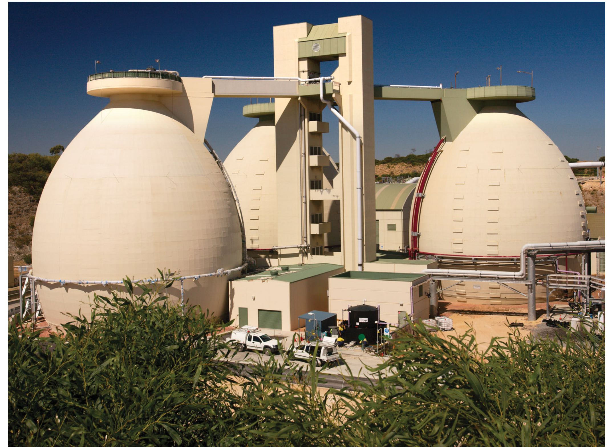
Digesters produce biogas feed for Hazer
