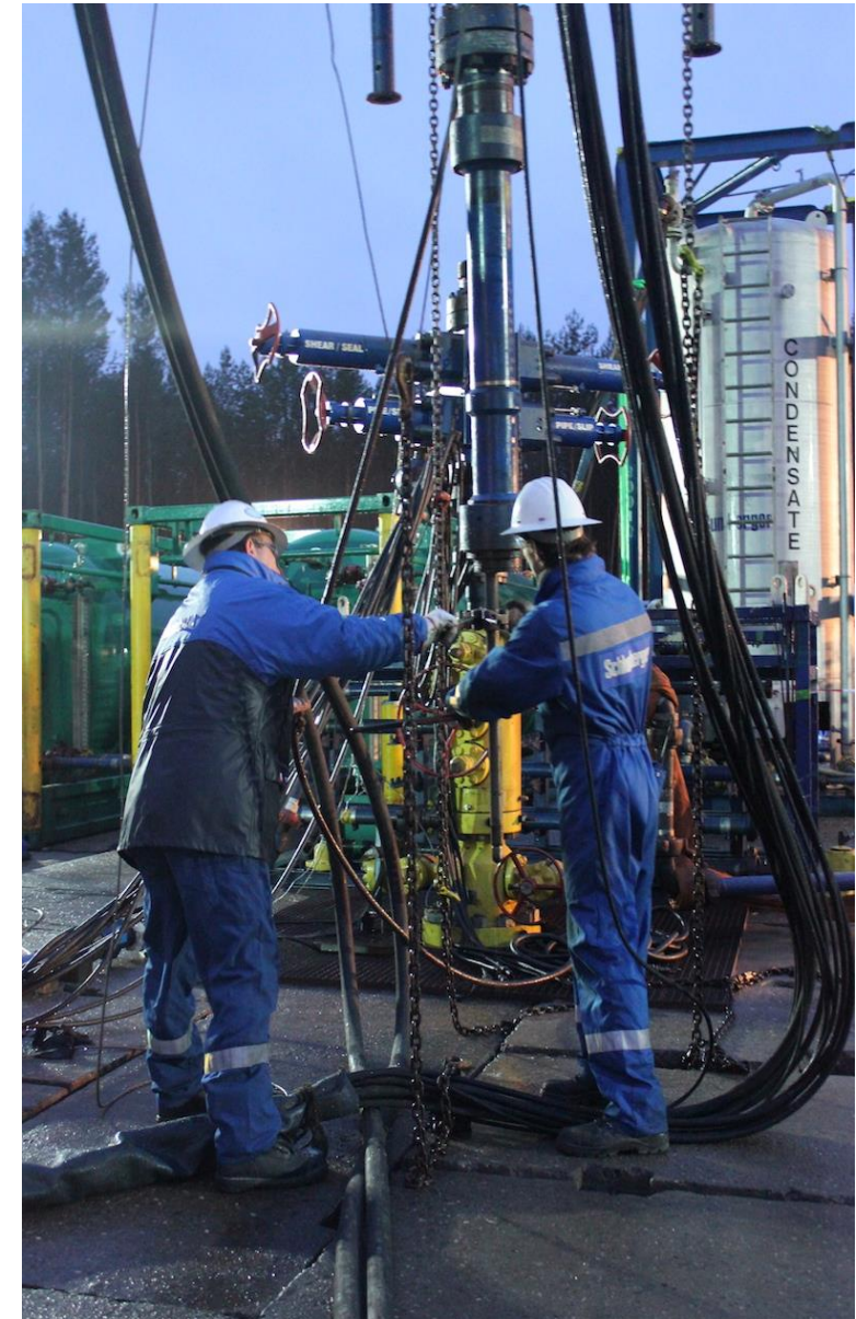
Photo: on location at Nowa Sol, Jany-C1
