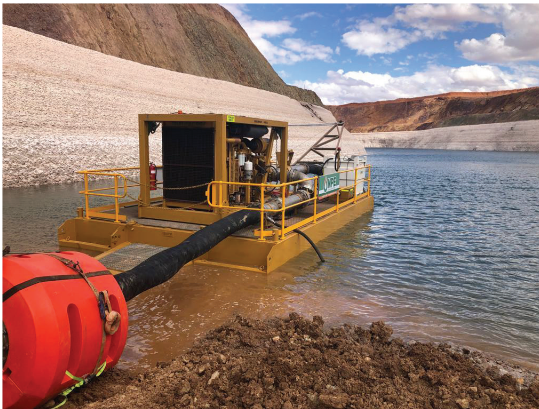
Figure 5: Dewatering of Williamson Pit
