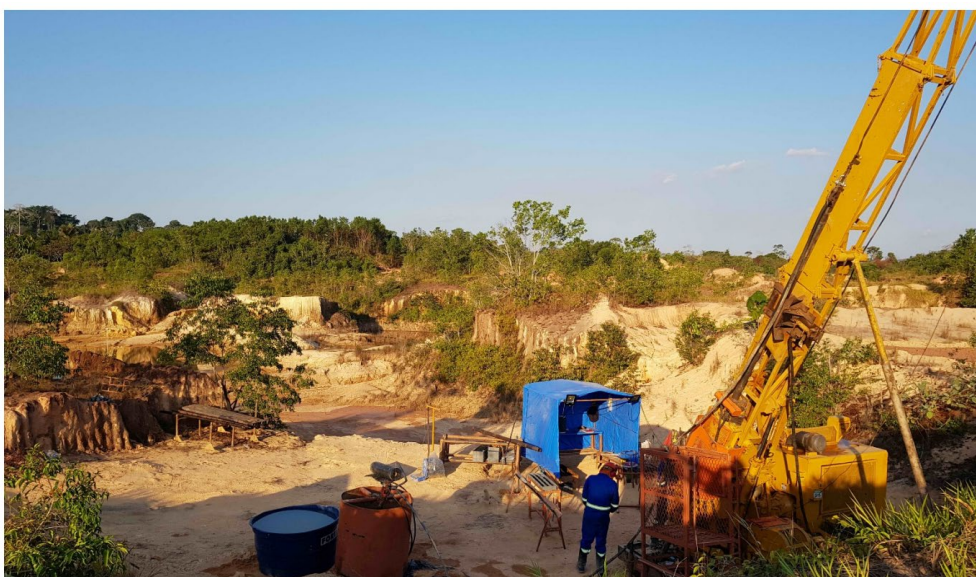
Figure 5: Drilling beneath the old workings at Dona Maria Prospect.
