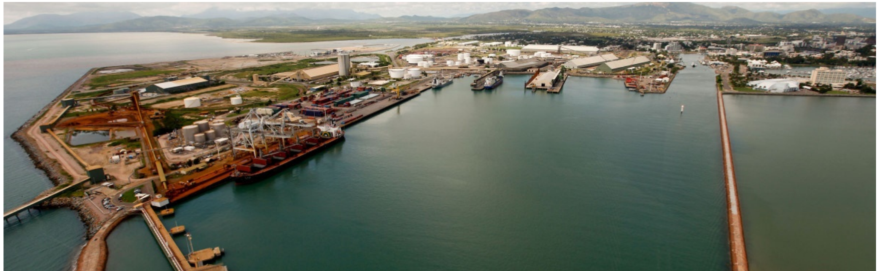
Figure: Port of Townsville
