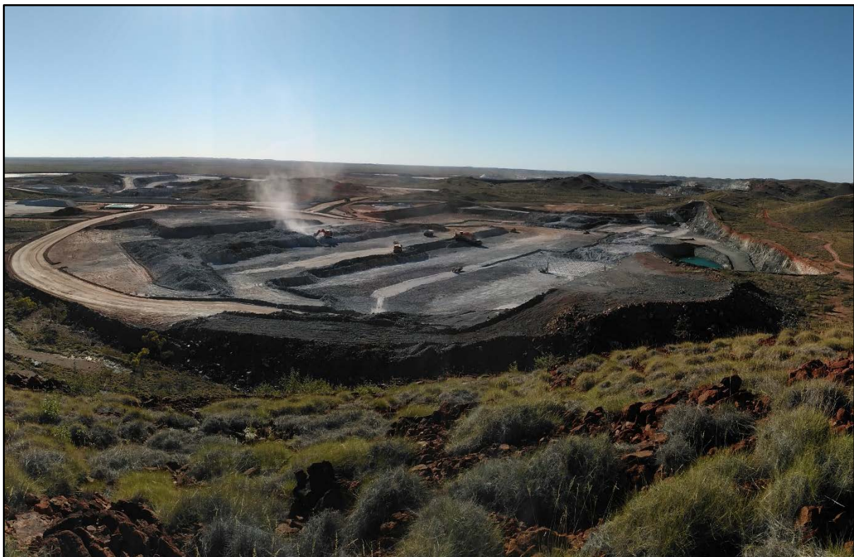
Figure 1 Mining Activities at the Altura Lithium Project – June 2019
