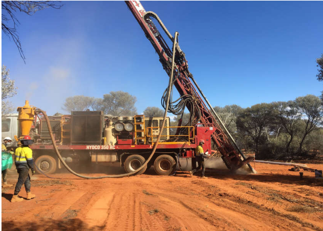
Figure 3: RC Drill Rig at Victory Bore
