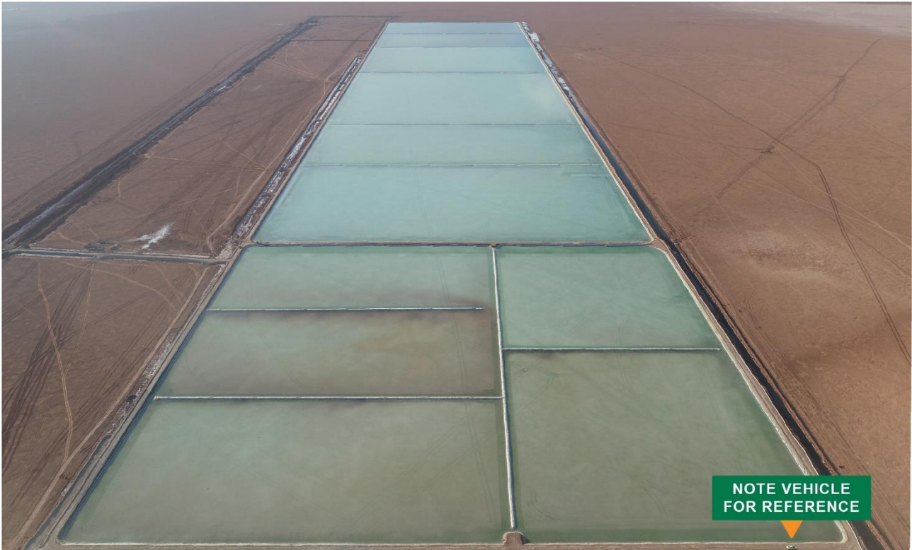
Figure 1: Completed solar evaporation ponds
