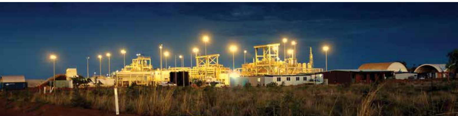
Above: Browns Range Pilot Plant.
