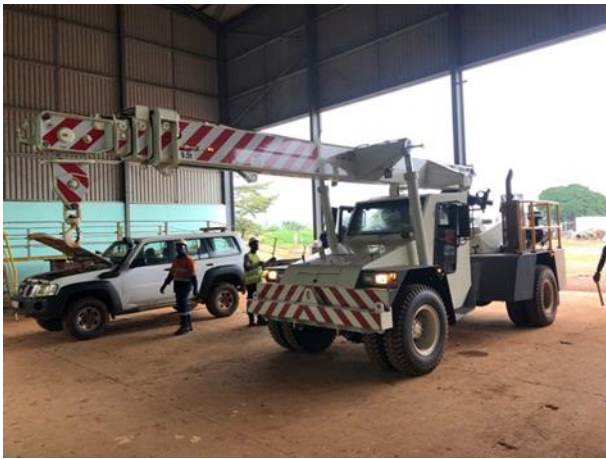
Franna Crane delivered to site
