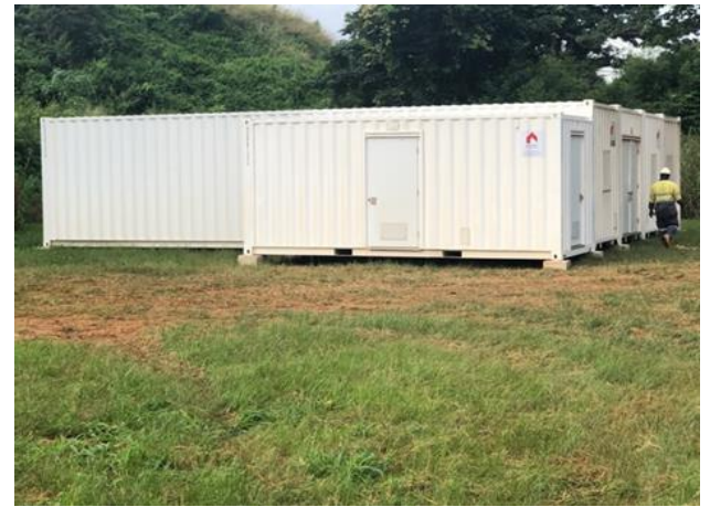
Temporary Accommodation blocks delivered to site
