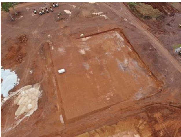
Switchyard building pad
