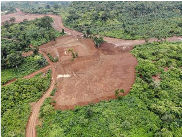
Construction Waste & STP areas
