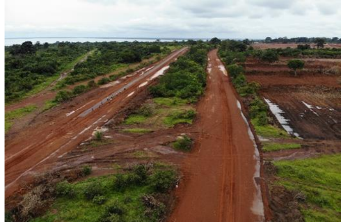
Fence installation towards Angovia
