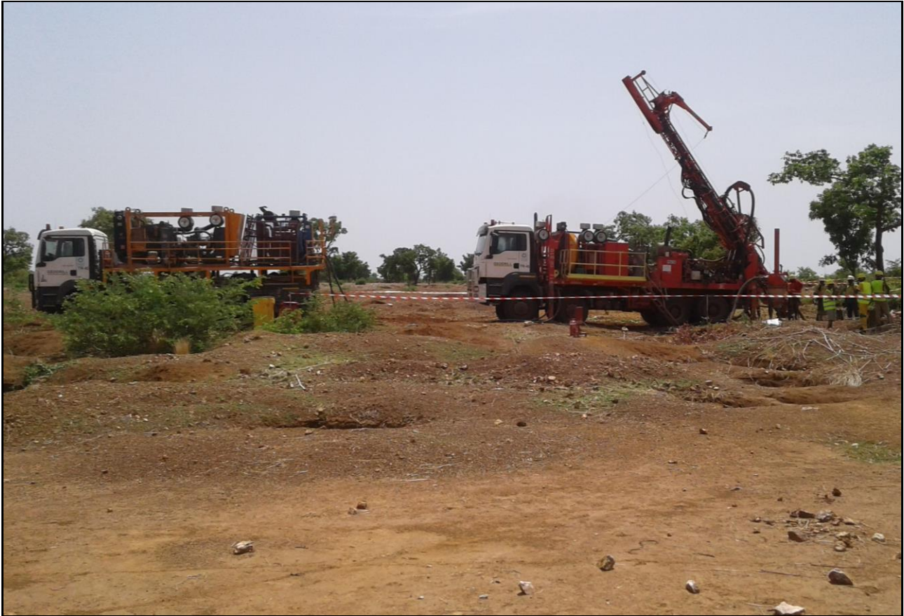
Figure 3: 2019 RC drilling programme at Divole East
