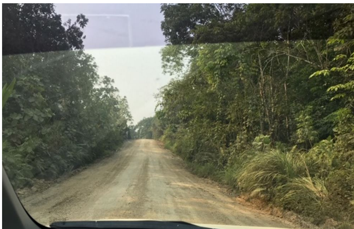
Logging road being used as a haul road
