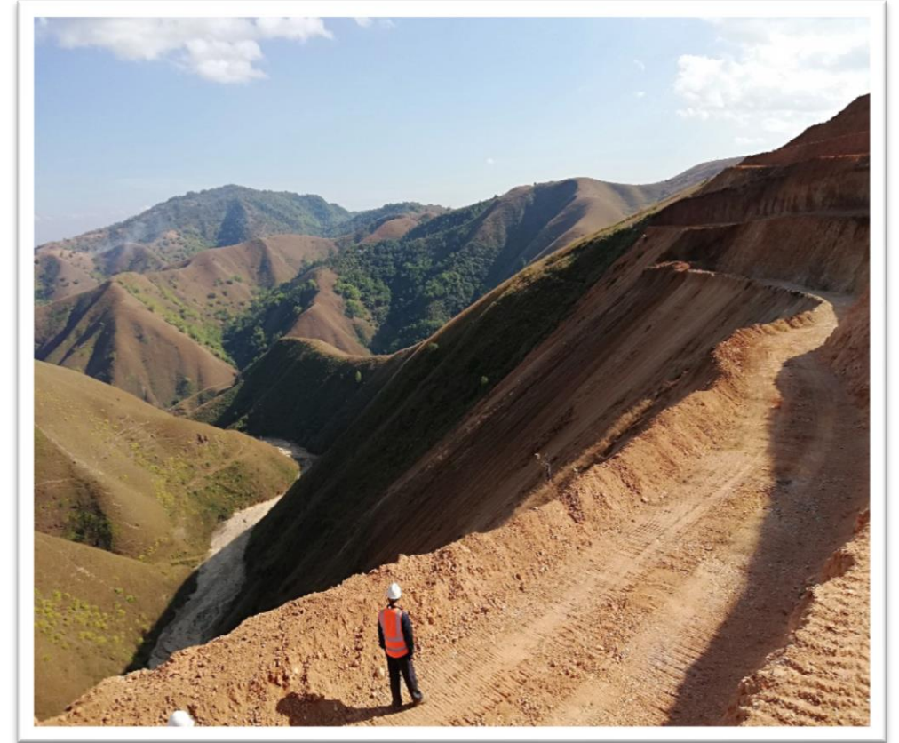
Drill access road to ER Valley
