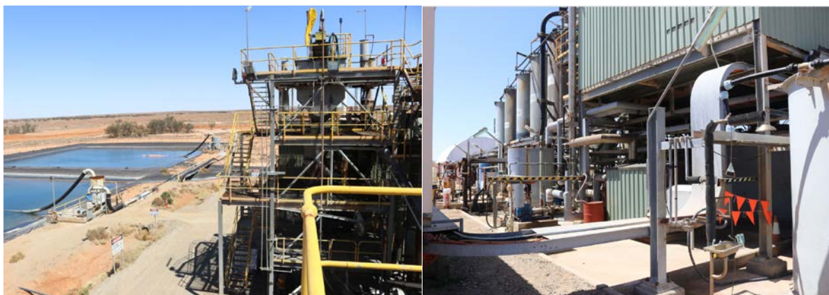
Figures: Existing Gold Recovery Plant
