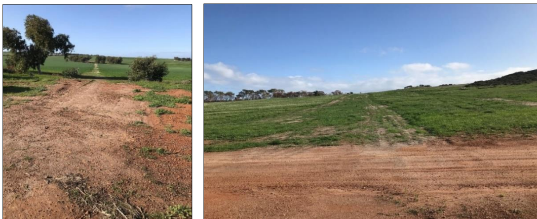
Flowline 8 from MH4 pad to MH8 pad (left figure), Flowline 8 (left lineament) and Flowline 4 (right lineament) (right figure). Rains have resulted in new grass germination along the length of backfilled sand
