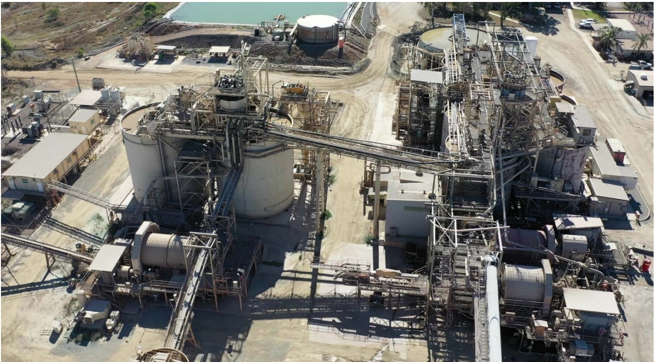
Figure 8: Nolans Processing Plant with third grinding mill (Mill #3) to be recommissioned to the left of picture. Existing grinding mills located in bottom right of picture
