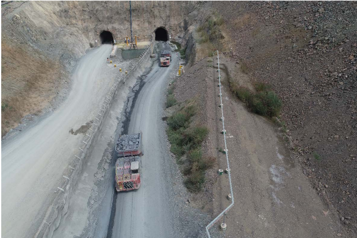
Figure 4: Automated Haul Trucks leaving the Syama Portal
