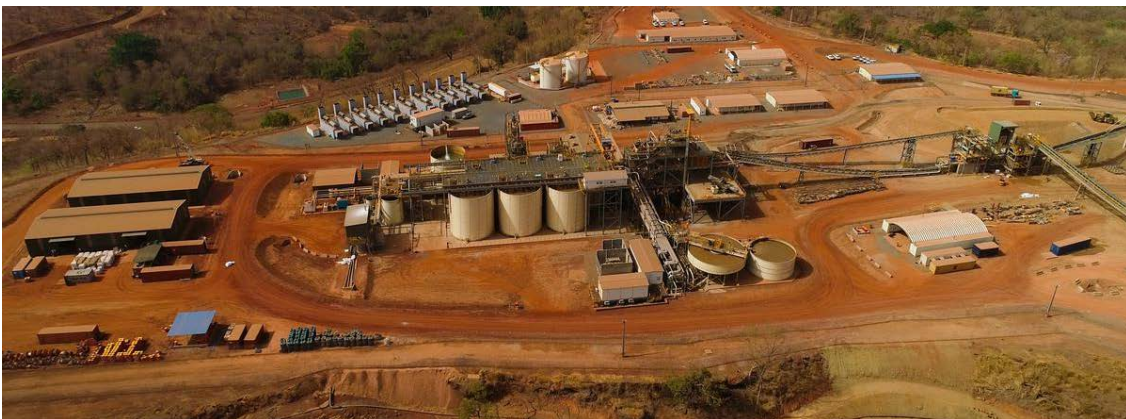
Figure 6: Mako Processing Plant
