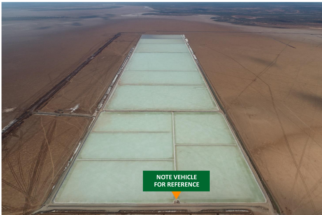
Figure 3: Completed solar evaporation ponds
